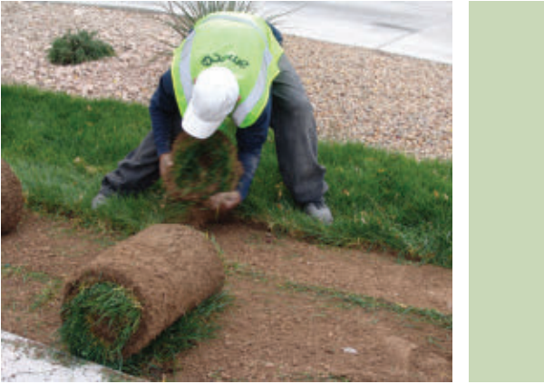
Southern Nevada landscaping crews remove grass in preparation for installing drip-irrigated water-efficient landscaping. Photo courtesy of the SNWA.
