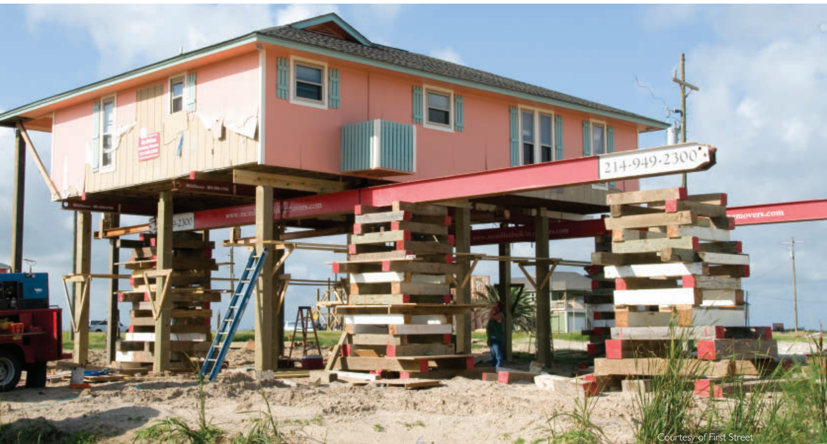
Courtesy of First Street
